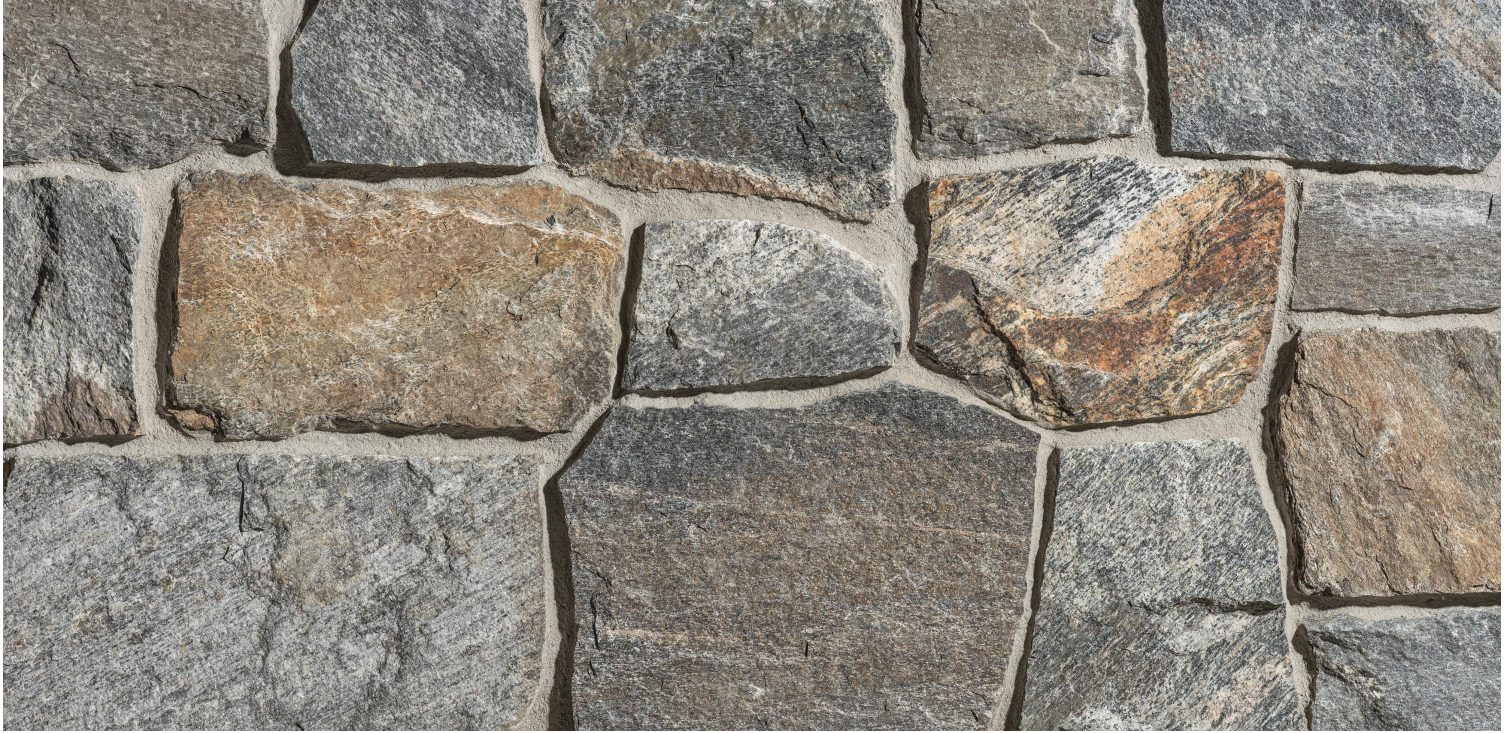
Photo Shows Installation With Mortar Joint
