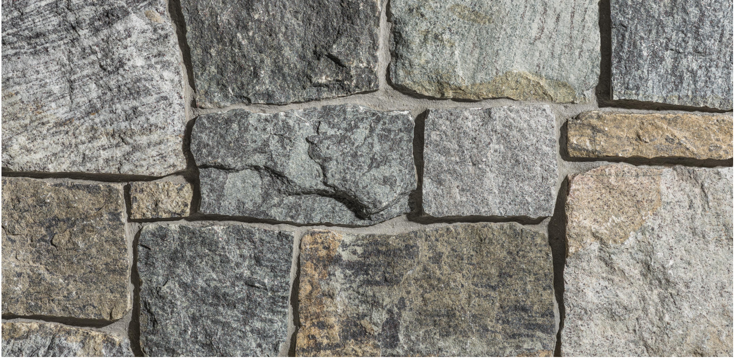
Photo Shows Installation With Mortar Joint
