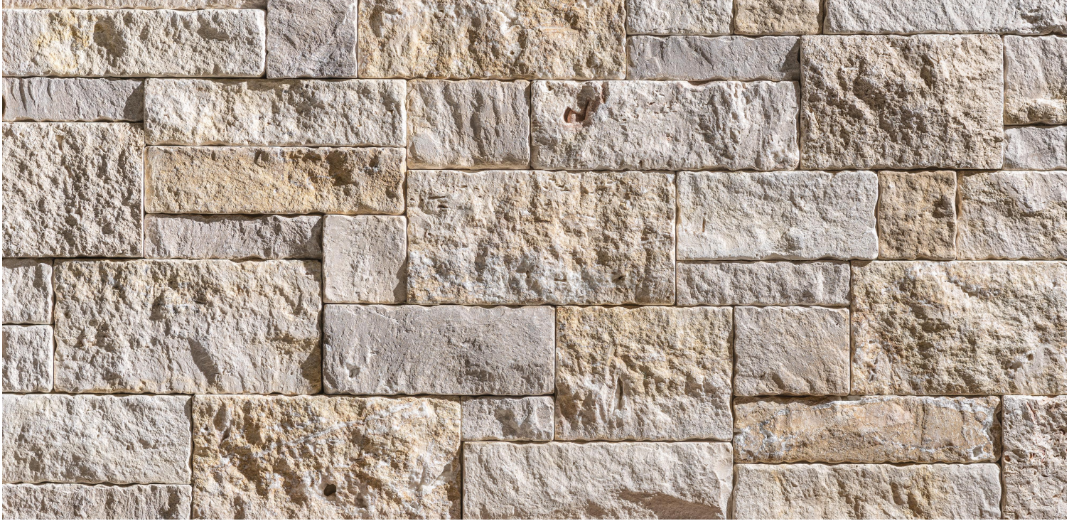
Photo Shows Dry-Stacked Installation
