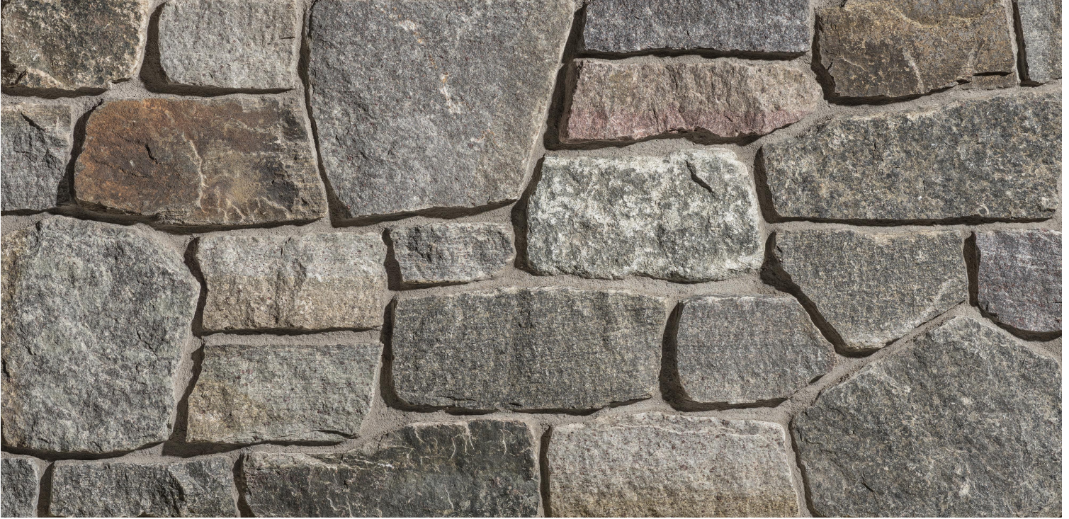
Photo Shows Installation With Mortar Joint
