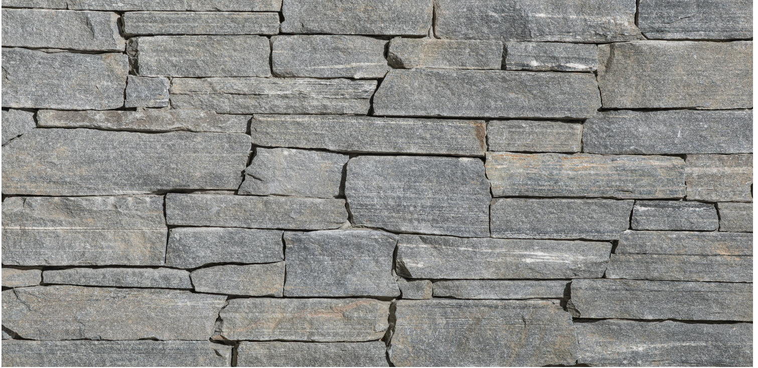
Photo Shows Dry-Stacked Installation
