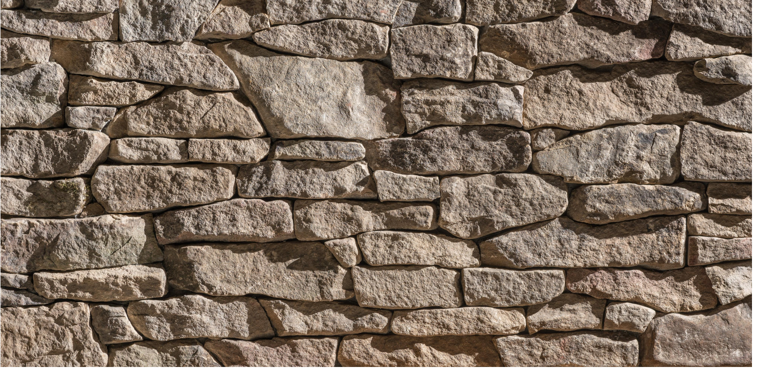
Photo Shows Dry-Stacked Installation
