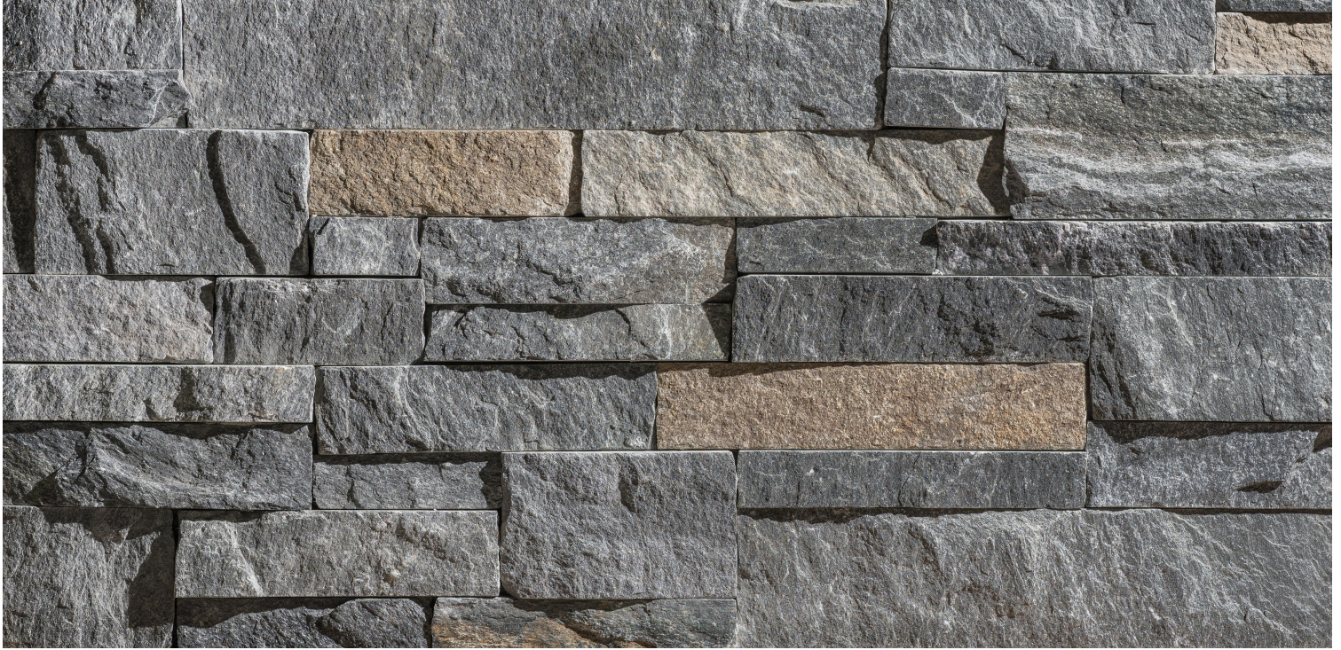
Photo Shows Dry-Stacked Installation
