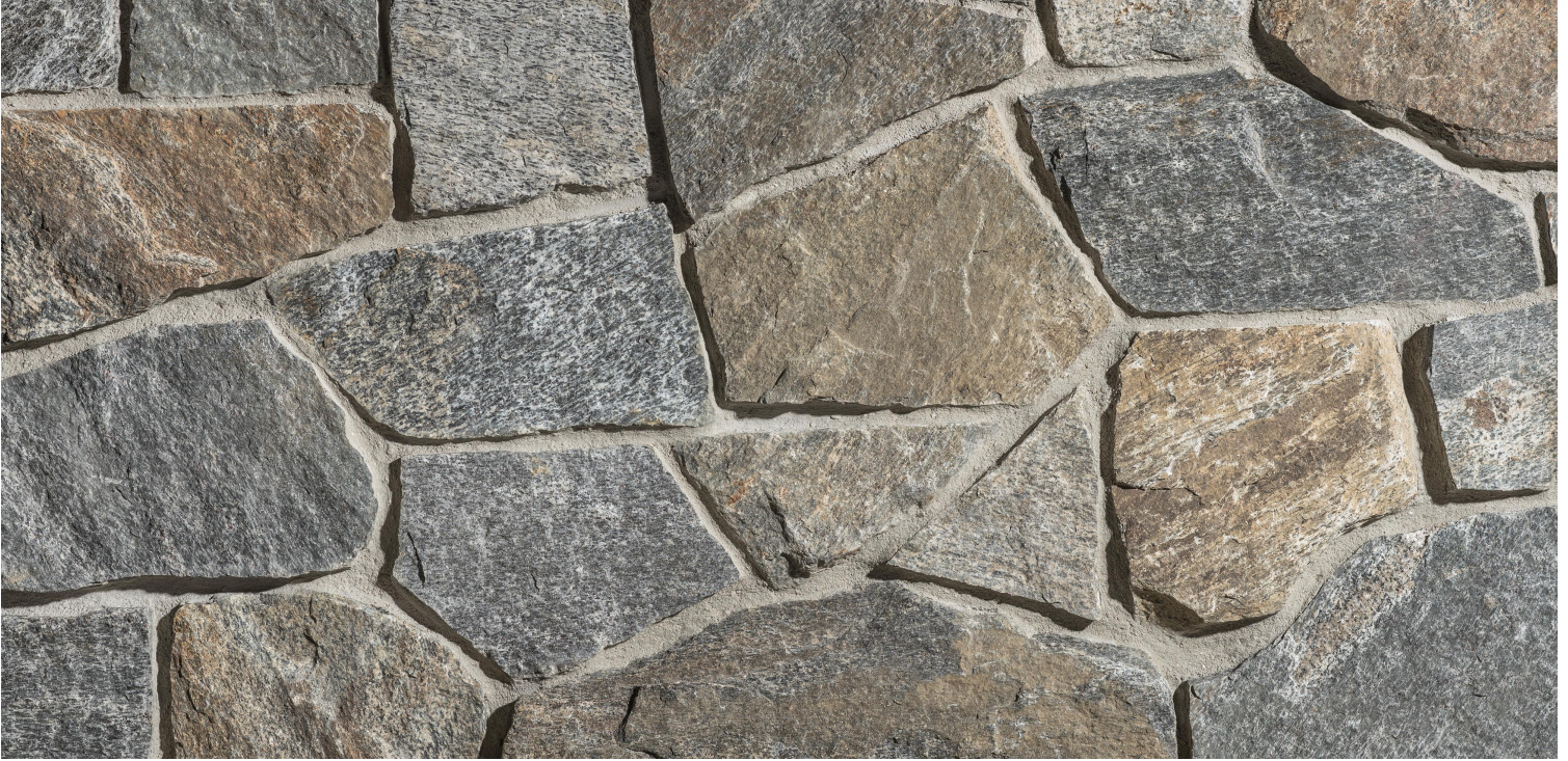
Photo Shows Installation With Mortar Joint
