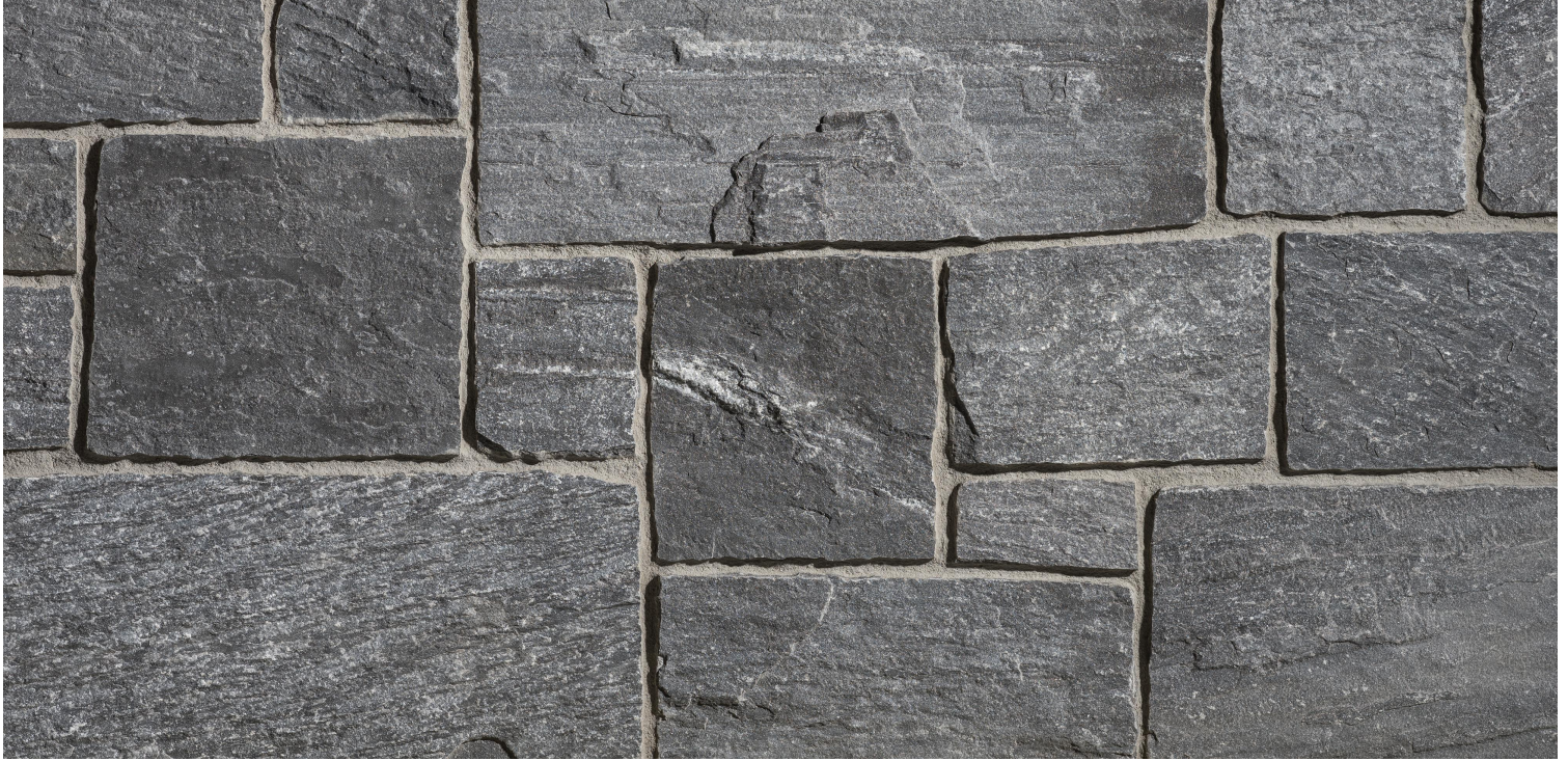
Photo Shows Installation With Mortar Joint
