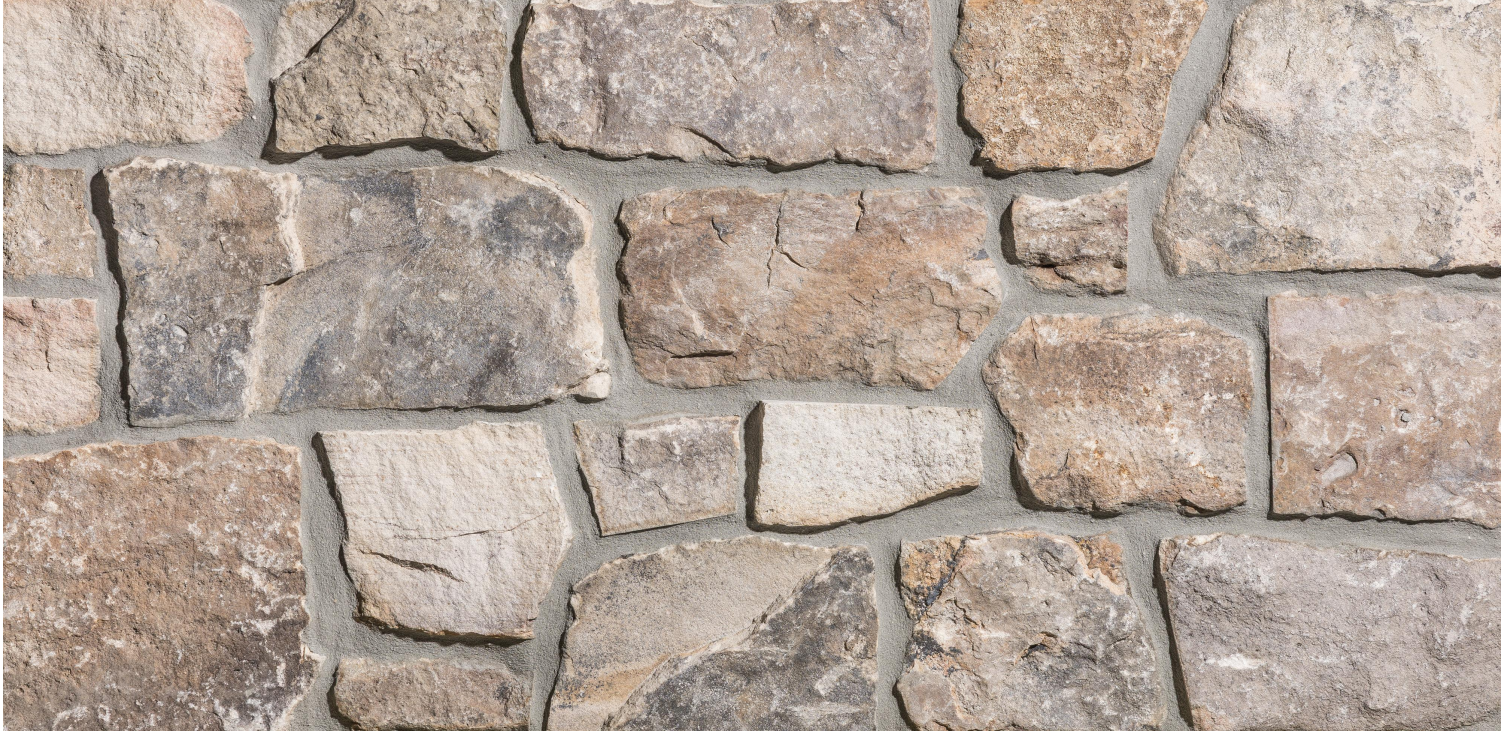
Photo Shows Installation With Mortar Joint
