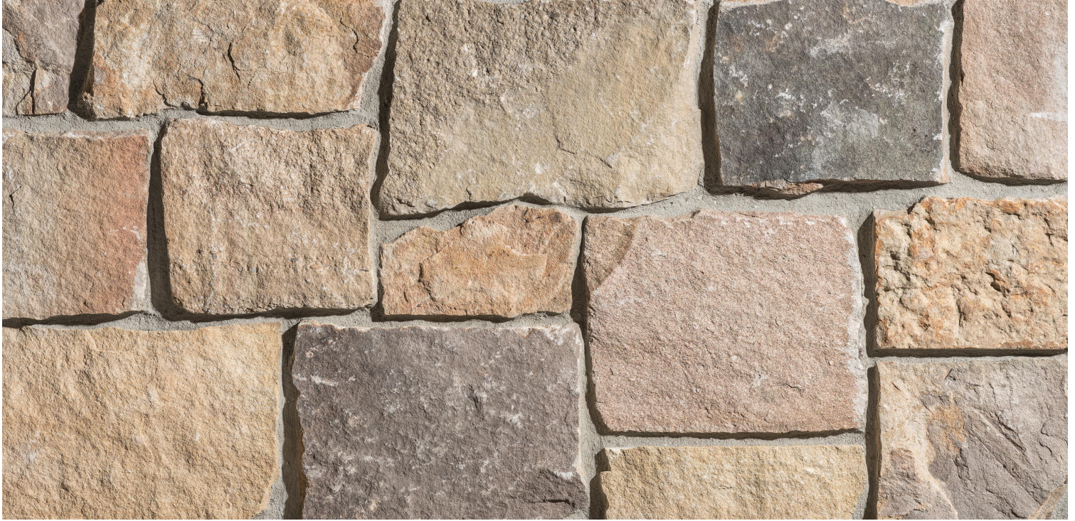
Photo Shows Installation With Mortar Joint
