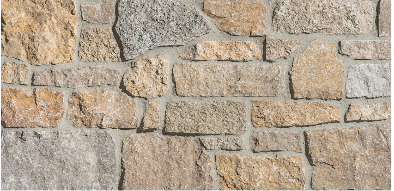
Photo Shows Installation With Mortar Joint
