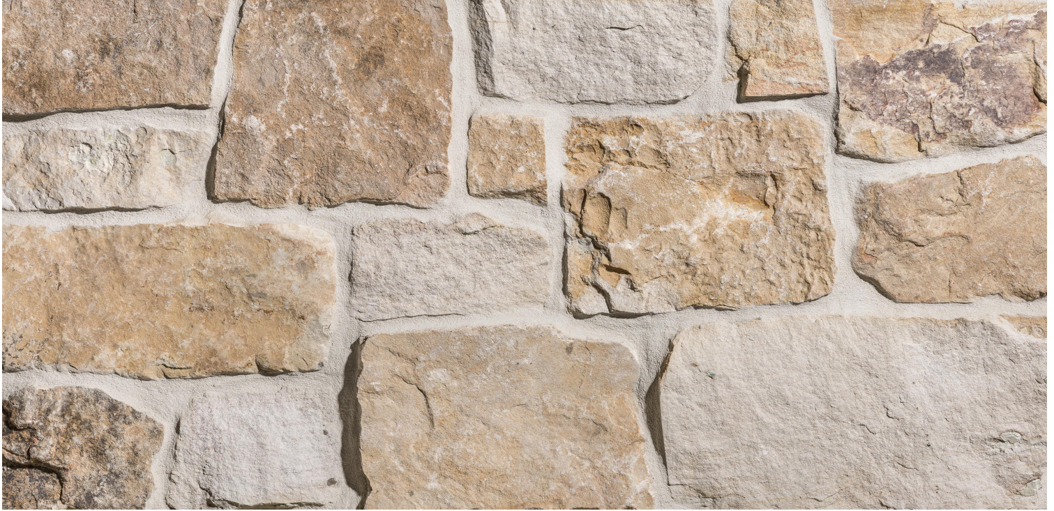
Photo Shows Installation With Mortar Joint
