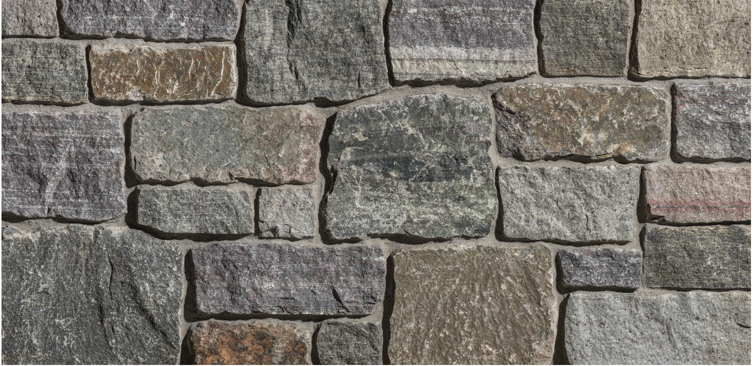
Photo Shows Installation With Mortar Joint
