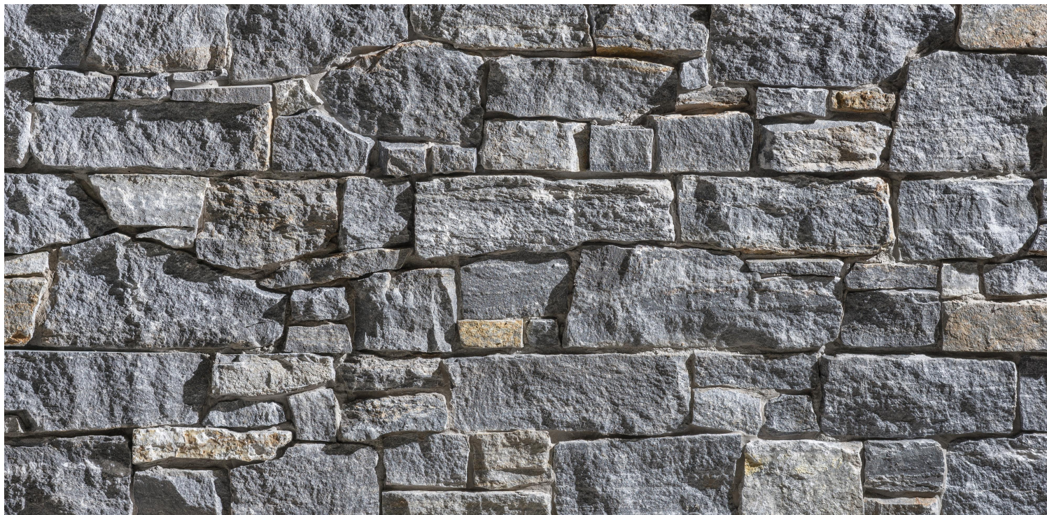
Photo Shows Dry-Stacked Installation
